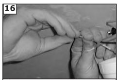
Make wire connections to power source using wire nuts provided. Make sure that no filiments are outside of the wirenut. After making the wire connections, the wires should be spread apart with the grounded conductor and the equipment-grounding conductor on one side of the outlet box and ungrounded conductor on the other side of the outlet hox.
